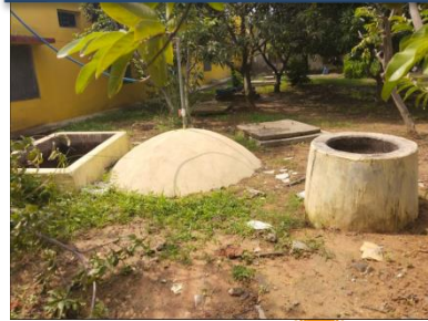
Kitchen food waste biogas plant
